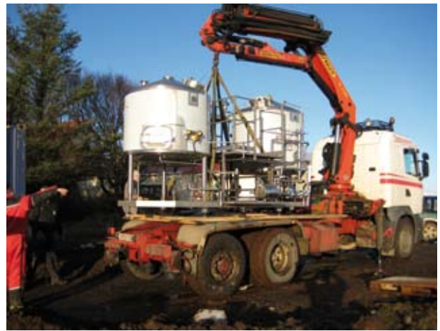
Transporting the brewhouse from a 40 foot container into the building.
